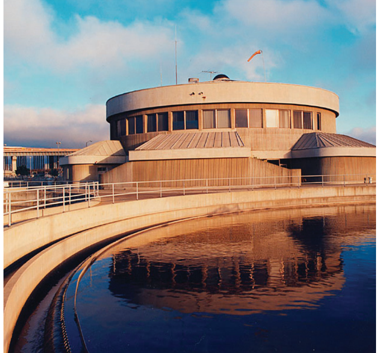
Settling tanks, big basins that hold wastewater, remove pollutants by collecting materials that naturally fall to the bottom and skimming off those that float to the top.
