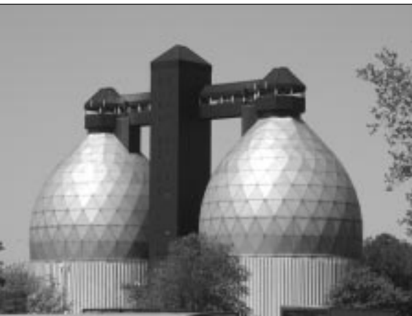
Back River Wastewater Treatment Plant
