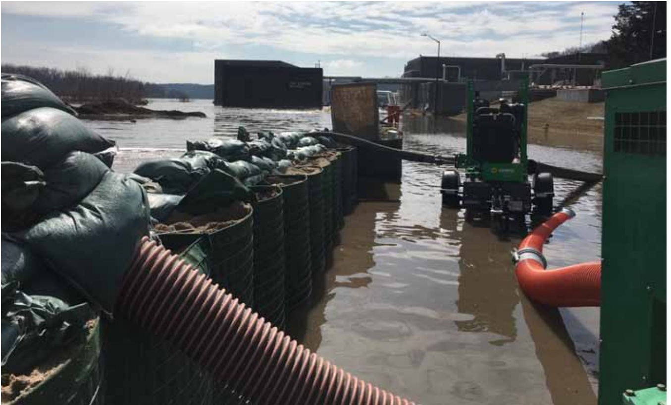
T o maintain primary treatment processes, operators at the Missouri River Water Resource Recovery Facility built a barrier of HESCO baskets in the flood waters. These baskets are containers that are filled with sand to create a flood barrier. Once the barrier was in place, crews were able to pump the water out of the facility. Additional sandbagging efforts were performed to protect vital electrical and mechanical facilities during the flooding. City of Omaha Public Works Department
