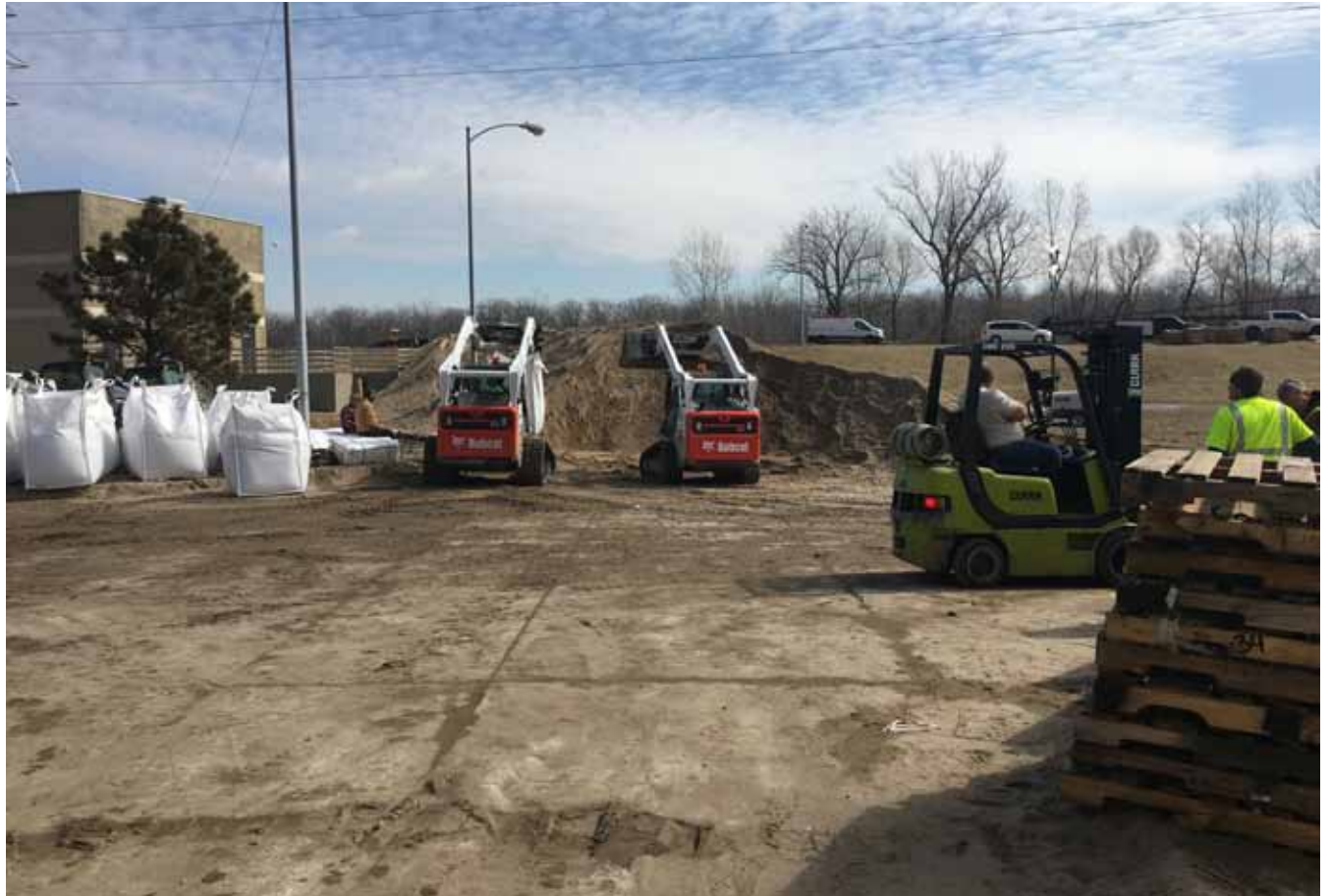
T o maintain primary treatment processes, operators at the Missouri River Water Resource Recovery Facility built a barrier of HESCO baskets in the flood waters. These baskets are containers that are filled with sand to create a flood barrier. Once the barrier was in place, crews were able to pump the water out of the facility. Additional sandbagging efforts were performed to protect vital electrical and mechanical facilities during the flooding. City of Omaha Public Works Department
