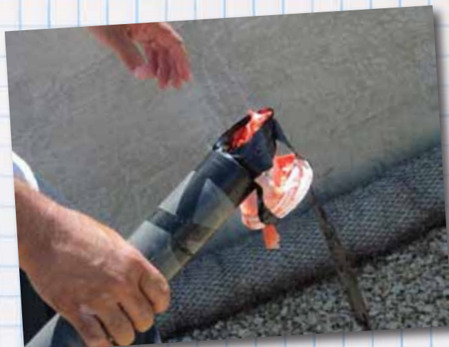
OPERATORS AT THE WESTERN MUNICIPAL WATER DISTRICT (RIVERSIDE, CALIF.) INVENTED A FEW SIMPLE DYE DELIVERY DEVICES TO QUICKLY TEST HOW ADDING NEW Baffles AFFECTED THEIR CHLORINE CONTACT TANKS. A SIMPLE COFFEE CUP AND LID TAPED TOGETHER AND SMASHED ON THE BOTTOM OF THE TANK WAS A GOOD STARTING POINT.
