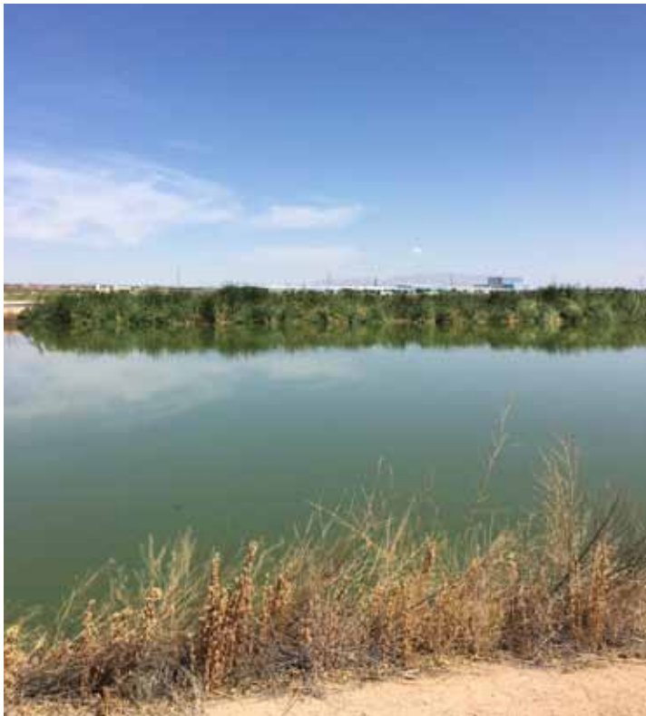
The facility's flow equalization pond and storage system provides for short-term storage of above-average flows due to normal daily flow variations. This allows for a consistent influent flow. El Paso Water
