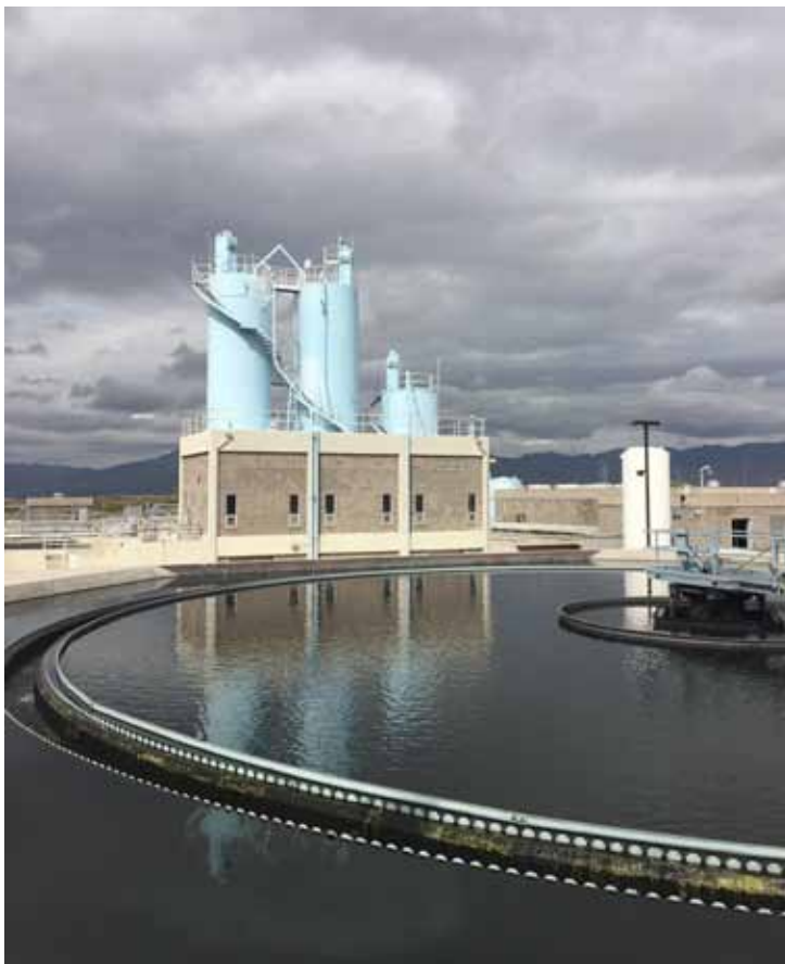
The facility's flow equalization pond and storage system provides for short-term storage of above-average flows due to normal daily flow variations. This allows for a consistent influent flow. El Paso Water
