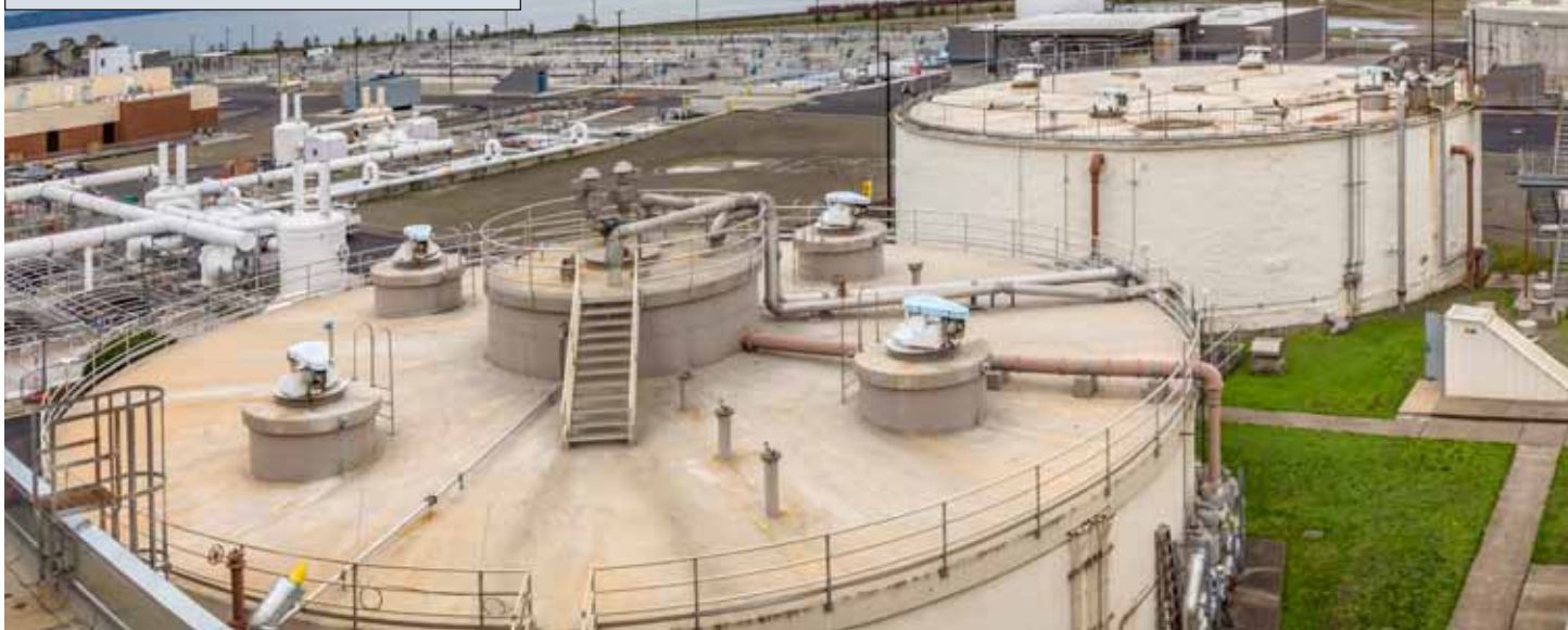
The upgrade of the Chambers Creek treatment facility was the single biggest public works project ever undertaken by Pierce County. The total project value totaled approximately $350 million. Construction of the new anaerobic digesters (shown) will provide solids handling capacity through 2040.
