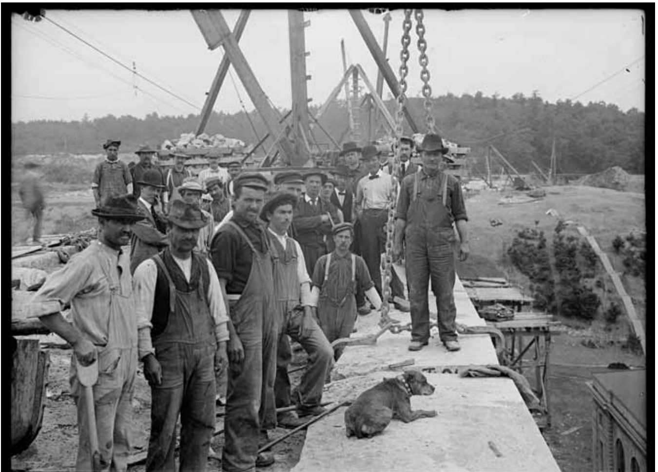
WACH. DAM, CLINTON, LAYING THE LAST STONE, JUNE 24, 1905.
