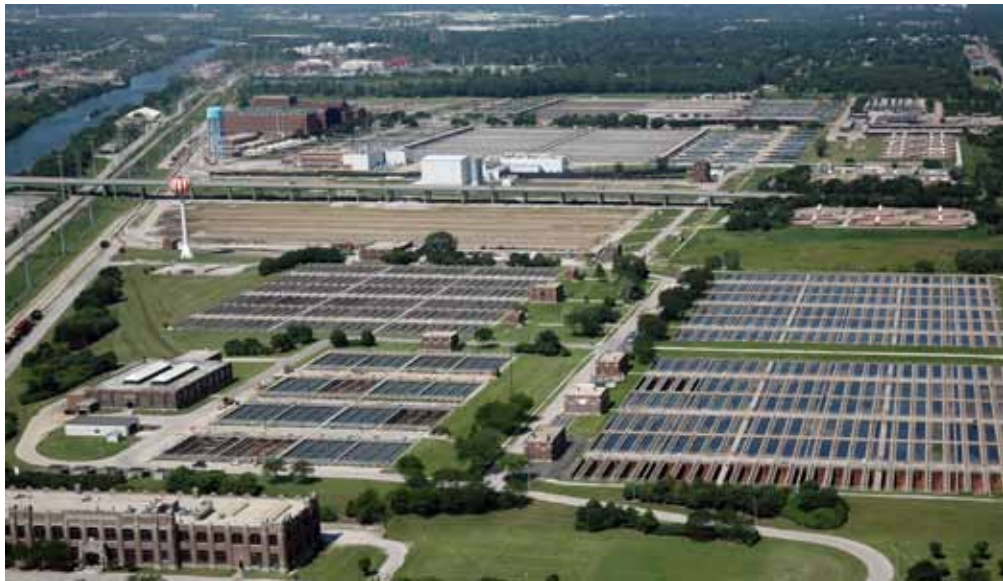
The 4.5-million-m 3 /d (1200-mgd) Stickney Water Reclamation Plant, near Chicago, is the largest wastewater treatment facility in the world. It serves 2.38 million people in a 673-km 2 (260-mi 2 ) area, including the central part of Chicago and 43 suburban communities. Metropolitan Water Reclamation District of Greater Chicago
