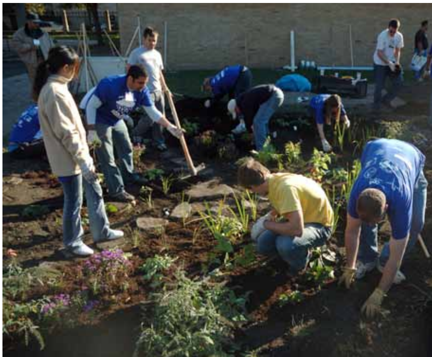
In addition to “gray” methods – capturing and containing overflows in pipes and tanks for later treatment – cities nationwide also began using such green infrastructure practices as rain gardens, bioswales, permeable pavement, green roofs, and more. Here volunteers plant a rain garden in Chicago during WEFTEC® 2008 in Chicago. Metropolitan Water Reclamation District of Greater Chicago
