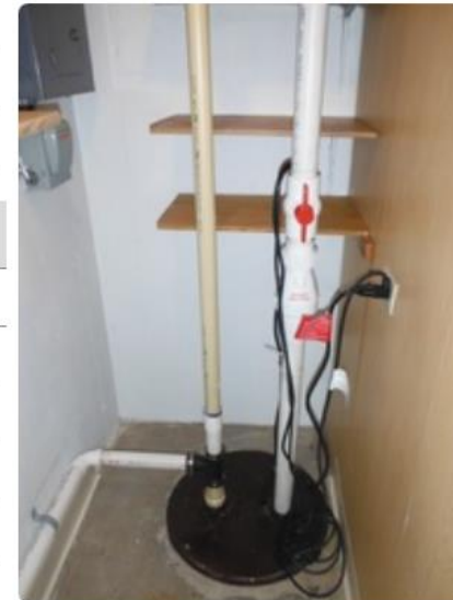
Pipes - Storm Sump
