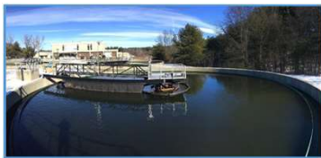
Marlborough Easterly WWTP, MA
