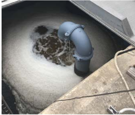
Centrate Equalization Tank
