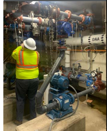
Rotary Lobe Pump for Centrate Feed
