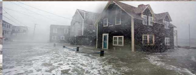
Homes on Lighthouse Road, Scituate, MA flooded by the March 2, 2018 Nor'easter. Photo: Channel3000.com
