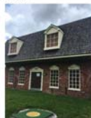
Photograph 31: PS 536 Front façade of building and manhole
