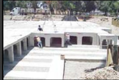
Construction of 1.7 acre infiltration chambers which are 5
