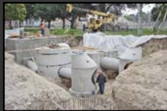
Installation of water treatment system at Sun Valley Park
