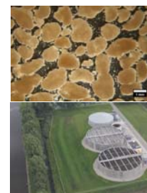
Nereda® Reactor at Gamerwolde WWTW
