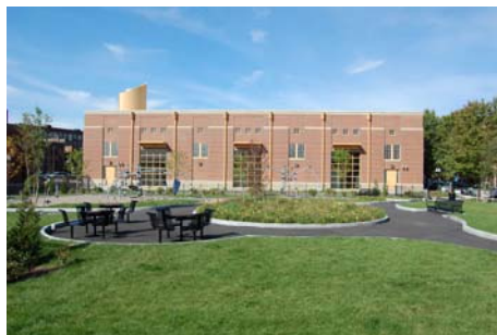
MWRA Union Park Detention/Treatment Facility
