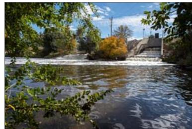
RWHTF outfalls, October 2014
