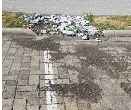
Localized sand accumulation, evidence of flow from upgradient roadway
