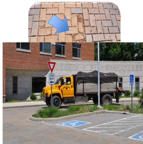
Cause of failure - siting
