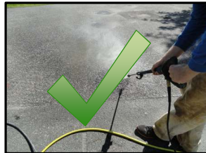
Pressure Washing (Porous Asphalt)
