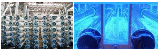
Additional RO/AOP Treatment
