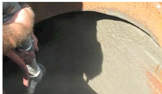
Gun Spraying Cement
