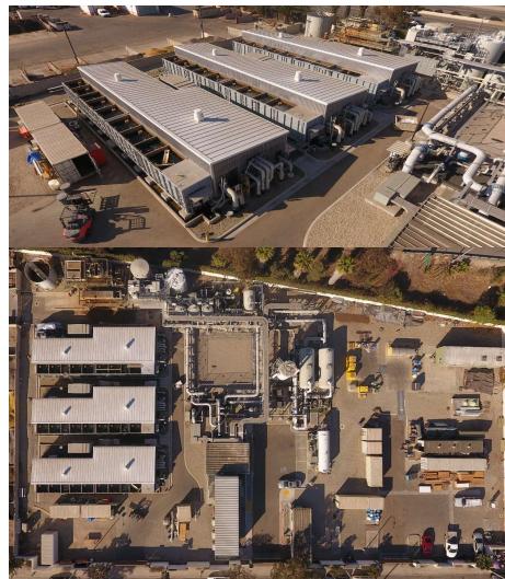
Charles Meyer Desalination Plant, Santa Barbara
