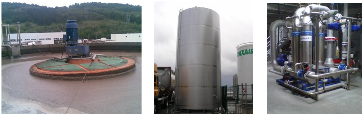
Figure 1. The biological reactor with the mechanical HPO injection aeration tank (left), equalization tank (center) and the membrane system (right).
