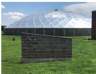
The Rapid City Water Reclamation Facility, located along Rapid Creek east of the city, may get $26 million in upgrades to maintain capacity and quality. (Photo: Bart Pfankuch)
