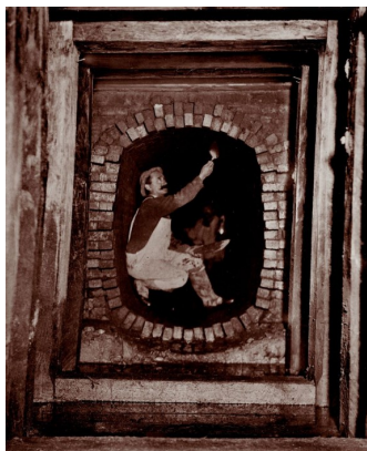
A man mortaring a sewer wall in 1880s Boston. (Photo: Boston Public Library)
