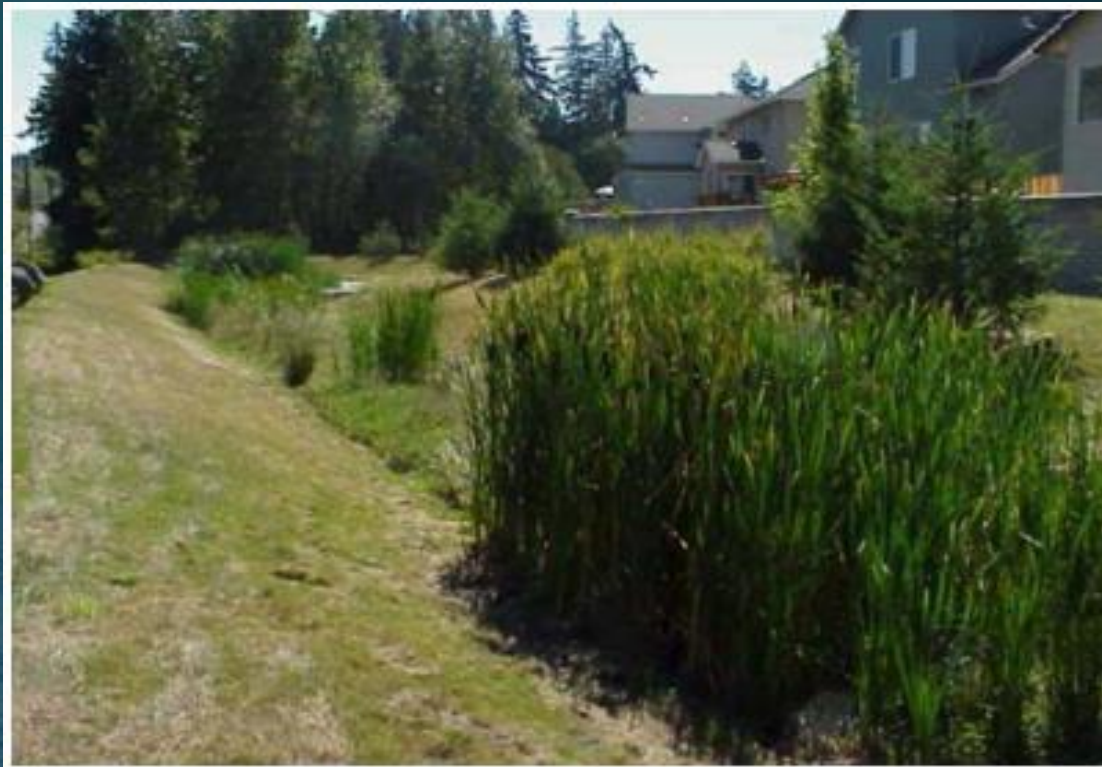
Figure 13: Example of a Vegetated Swale
