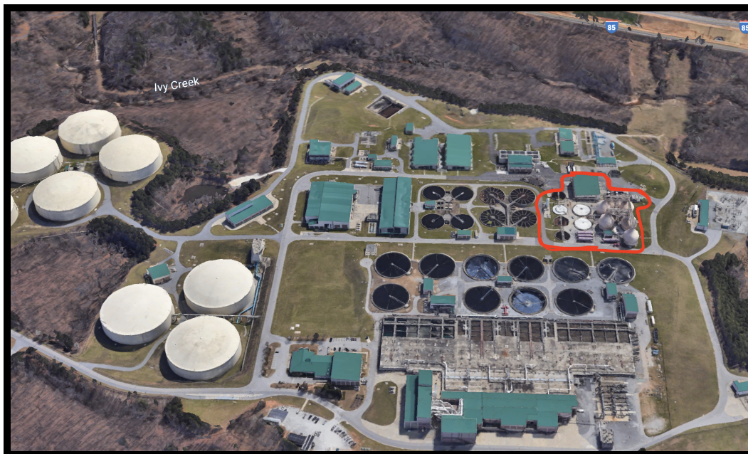
Figure 1. Aerial photograph of F. Wayne Hill Water Reclamation Center (FWHWRC) with the solids handling treatment train outlined in red.
