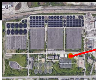
O'Brien Water Reclamation plant, Skokie, IL
