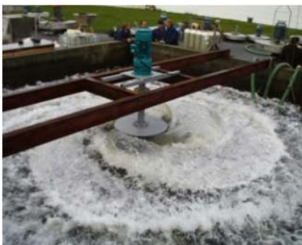
Figure 1—Radial flow low speed surface aerator [2].
