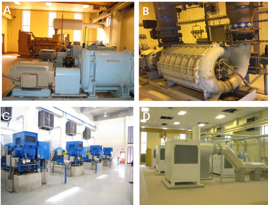
Figure 1— Different Blower Types – (A) Positive Displacement (Rotary Lobe), (B) Multistage Centrifugal, (C) Single-Stage Integrally Geared, (D) High Speed Direct Drive (Turbo)
