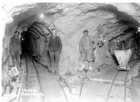
Figure 3 – Photo of workers constructing a connection between two sewer segments in an underground chamber of MWRDGC's Salt Creek Tunnel.
