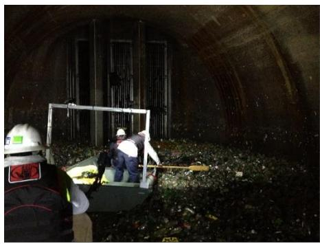
Figure 11 – Photo of operations staff removing floatables from a tunnel at Milwaukee MSD.
