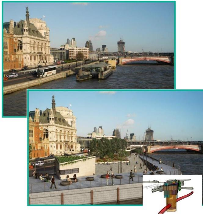
Figure 7 – Before and after for the Blackfriar drop shaft location along the Tideway Tunnel. Thames Water utilized green infrastructure to provide both a community walkway and tunnel access for operations staff. (Photo's provided by D. Crawford)
