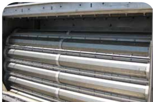
USA, California Eliminator™ Tertiary treatment, 2mm openings 20.7 MGD (78 MLD)
