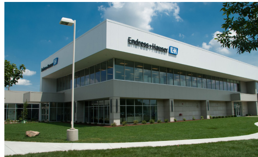
Endress+Hauser, Inc. Customer Center in Greenwood, IN
