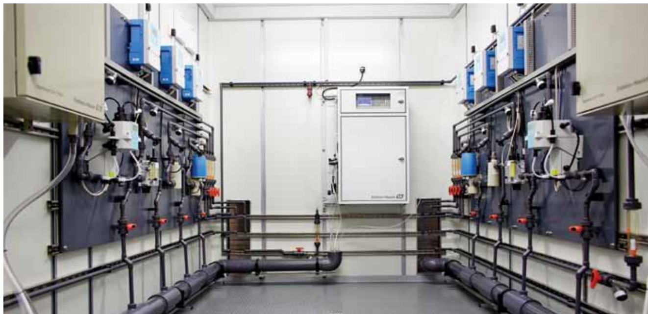
Container solution of Endress+Hauser for efficient water management in production and auxiliary circuits
