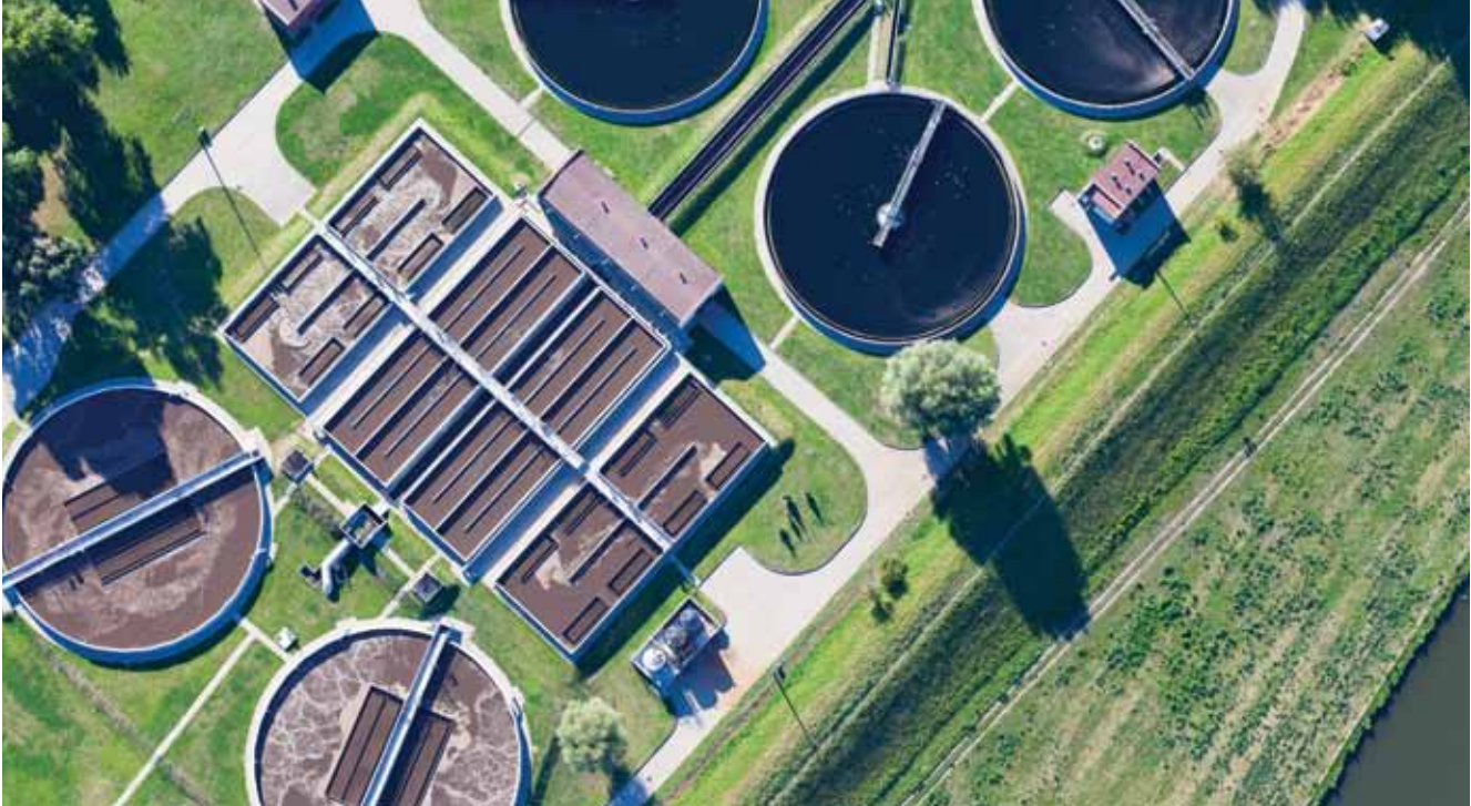
Modern sewage treatment plant that also meets strict requirements
