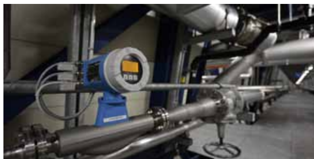
Coriolis-based density measurement in the sludge conditioning process with a Promass device
