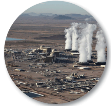
Palo Verde Nuclear Generating Station Water Reclamation Facility
